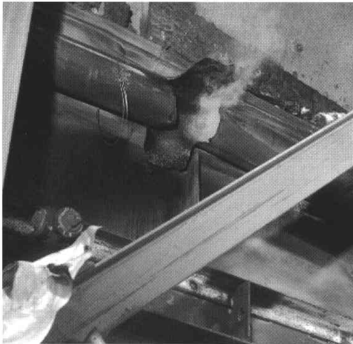
Six-inch boiler feedwater pipe rupture
