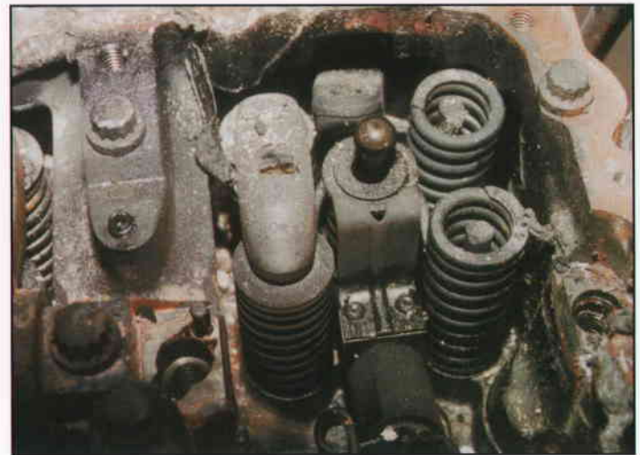
Photo 8 - Damaged Valve Components (South Engine)
