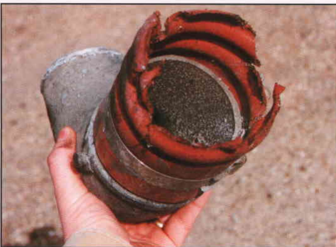
Photo 11a - Turbocharger Outlet Rubber Hose Connection Mechanical Failure (South Engine)
